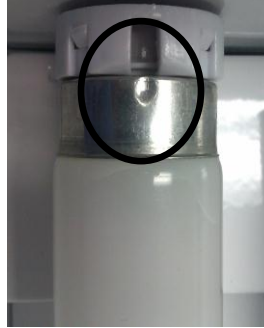
Diagram 1-T8 lamp seating
