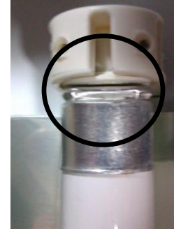
Diagram 2-T5 lamp seating
